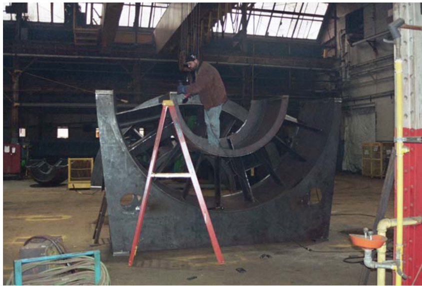
Figure 11: Arc-torch cut marks were ground smooth.
